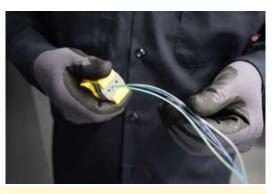
Align the fiber jacket or buffer tube to the proper channel
